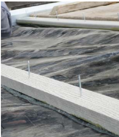
Tacking Strips and Rolled Mats Used on Previous Project.
