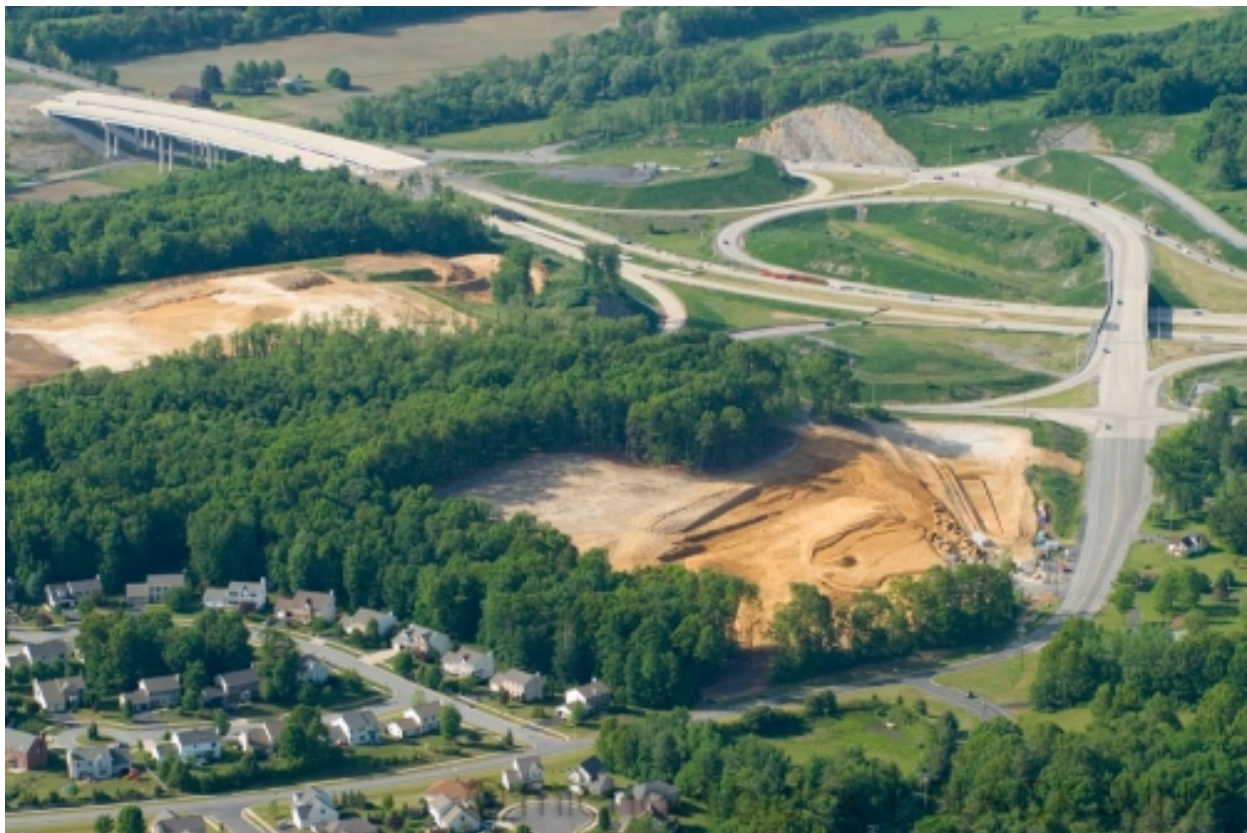
Aerial View of Gray's Woods Site off of US Route 220/322
