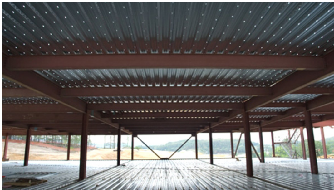
View from first floor of structural bays during construction.
